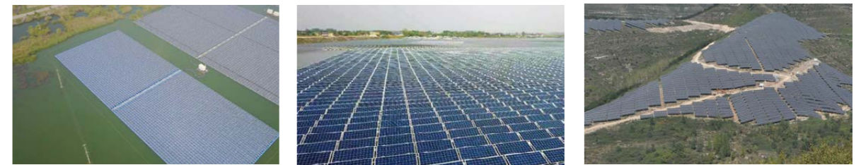
40 MW Floating PV Project in Huaibei, Anhui
