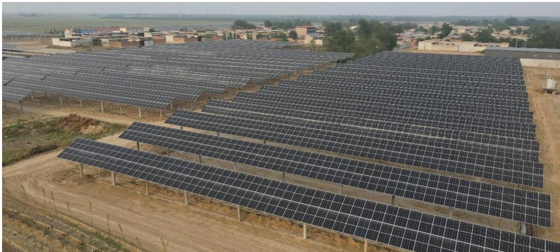
SuperTrack has been applied to 400MW project located in Nangong, China. The tracking system was connected to grid in June 2021. By the end of September, Tracking system had operated for 77 days, including 25 days of highly diffused irradiance weather, and the average power generation gain in highly diffused irradiance weather was 3.84%, including a typical cloudy day with a power generation gain of 8.03%.
