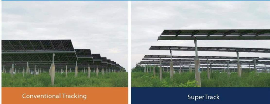
As shown in the figure 23, on overcast or rainy days, SuperTrack will place the tracker at a small angle or keep the tracker flat according to weather conditions. The greater the difference between the array angle of conventional tracking algorithm and the optimized array angle, the higher the gain of SuperTrack power generation. On typical overcast and rainy days, the daily power generation gain may reach 12.86%.
