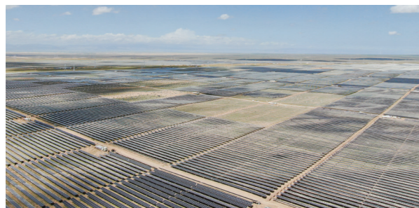
Figure 4: Yellow River Hydropower Qinghai High Voltage Power Station 135M project
