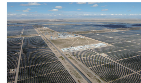
Figure 24: Yellow River Hydropower Qinghai Ultra-High Voltage Power Station 135MW Project
