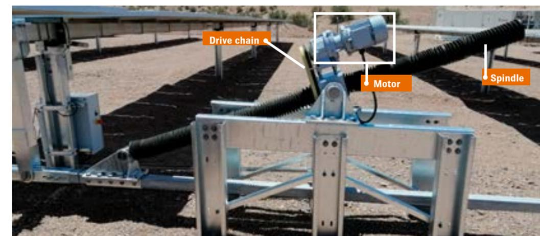
Note: The location of the indicated elements may vary according to the design of the tracker, but their functionality within the assembly does not change.
