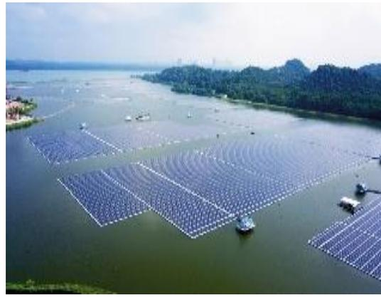
In August 2021, grid-connection of a Singapore 60MW photovoltaic project built with Trina Solar 210 Vertex Modules!
