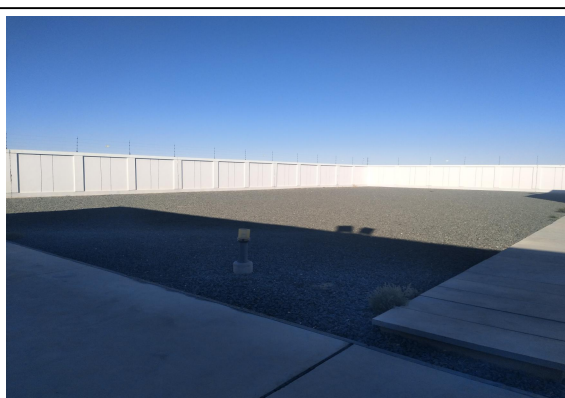
升压站内砾石压盖
