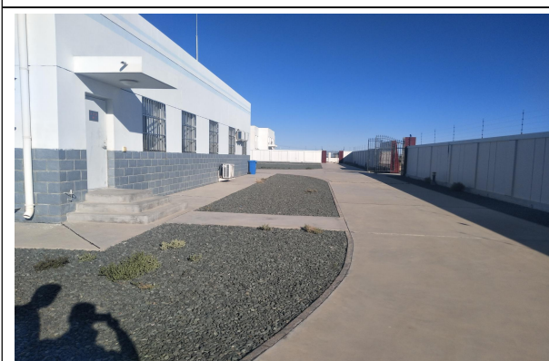
升压站内砾石压盖
